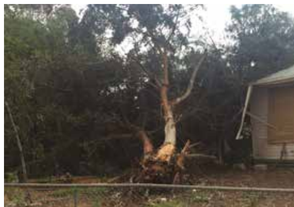
Significant damage revealed the day after the Mildura Storms. Courtesy of Emergency Management Victoria.
